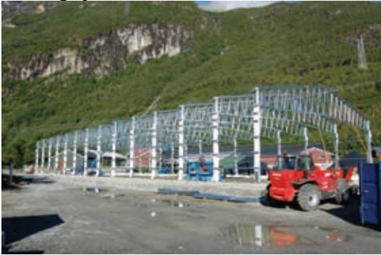
Framework constructions for the hall.
