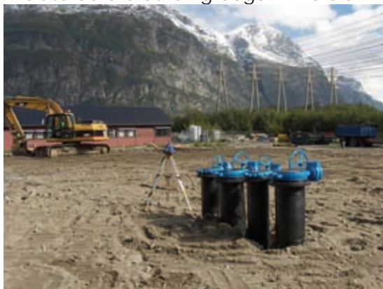
The levelled site with intake pipes in place.
