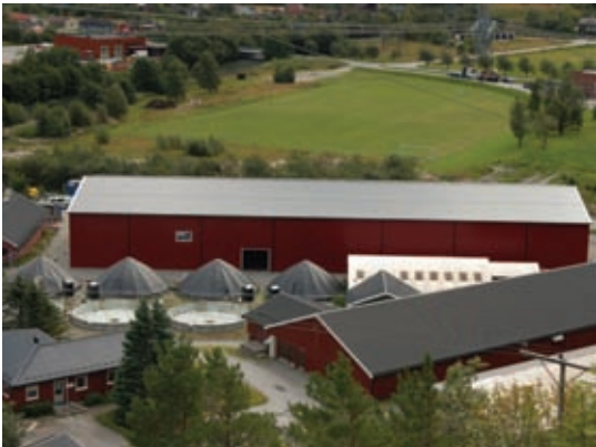
Main construction for the hall.
