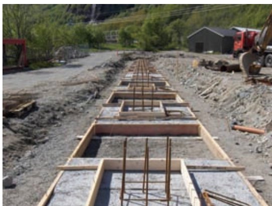
The foundations for the hall.
