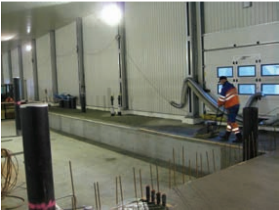
Concreting is completed in the central water treatment room.
