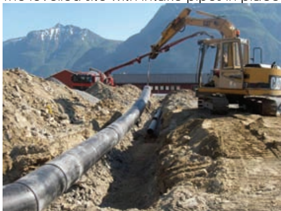
The main outflow pipes are placed in position.
